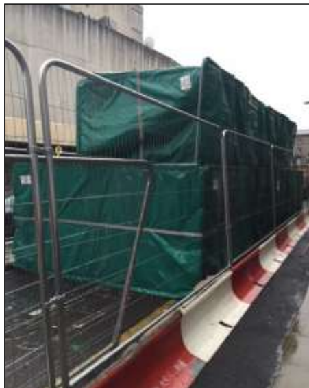
3 sided Acoustic enclosure for surrounding breaking, cutting works
