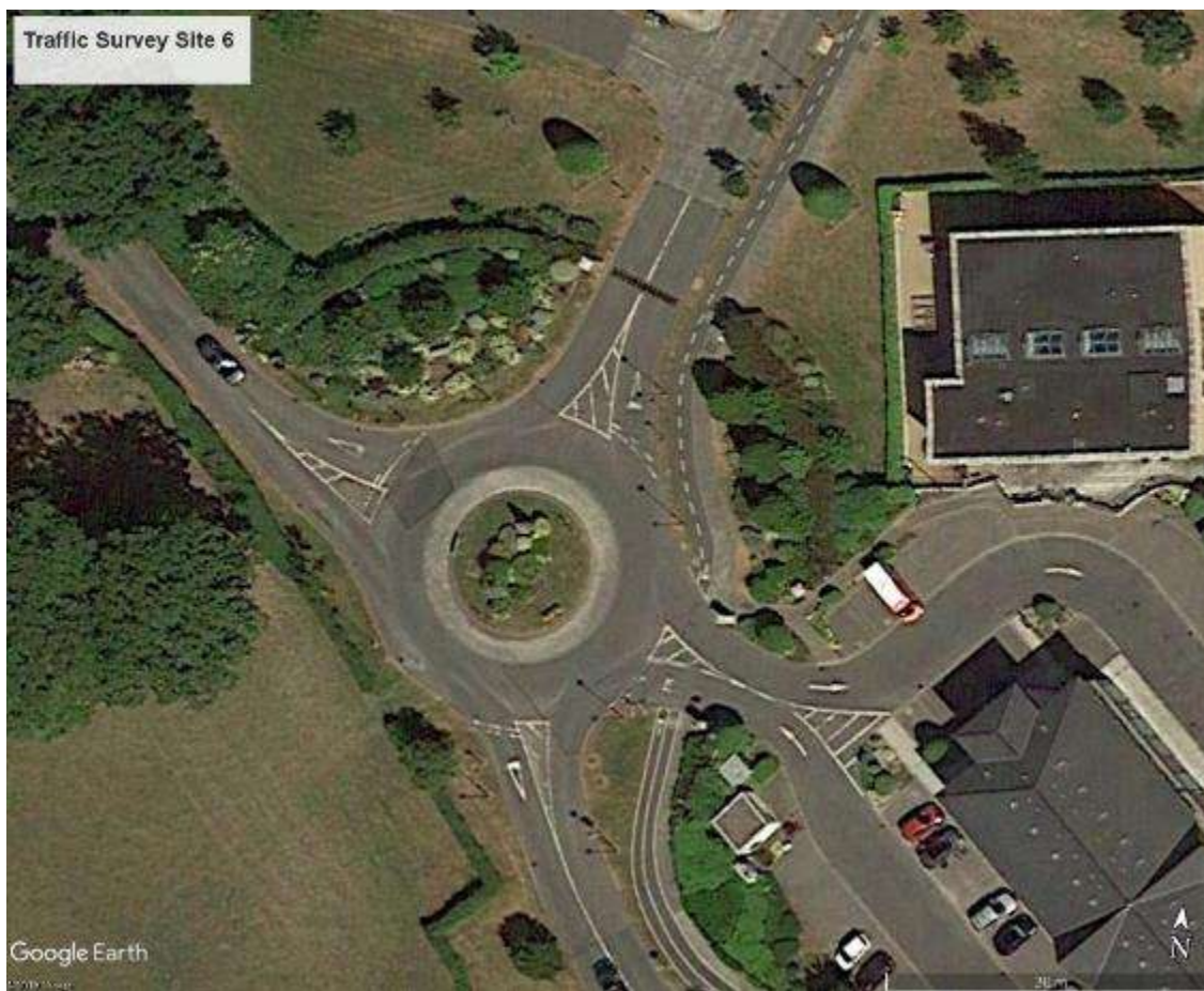
Figure 10.14 – Aerial Image of Eden Gate Roundabout
